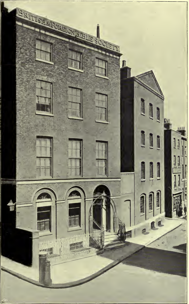
OLD BIBLE HOUSE, 10 EARL STREET.
